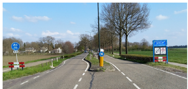
Image 8: Built-up area boundary not in accordance with BABW.
